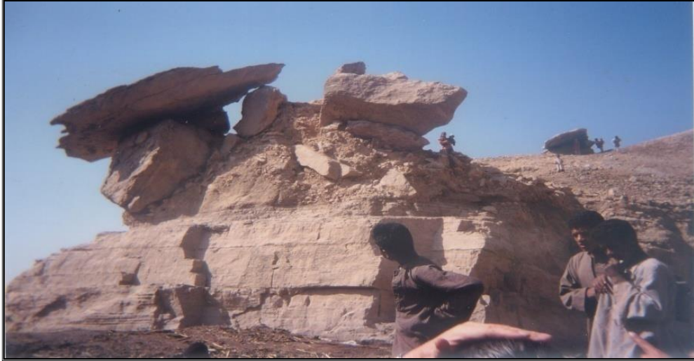
Photo 9. Blocks threatening to collapse (El-Mahamied)
