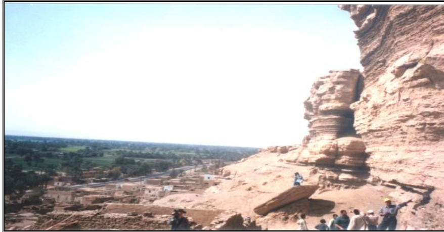
Photo 5. Crack cutting the slope of the embankment (El-Mahamied)
